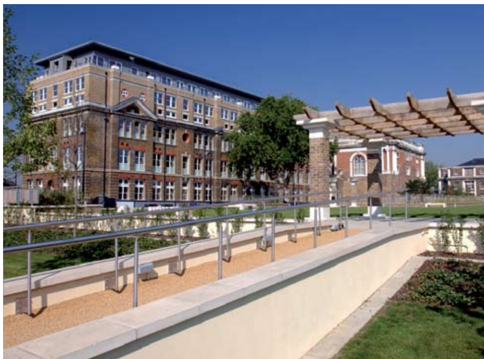
After taking control of the land in 2000, London Development Agency led on the planning and delivery of a new mixed use urban quarter at Royal Arsenal in this part of the Thames Gateway. Delivered by the preferred developer Berkeley Homes, the design quality of the first phase has been recognised through a Building for Life award in 2008
